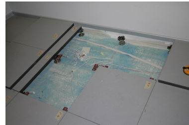
(b) Floor tiles rest on columns.
